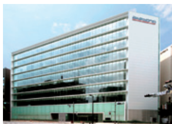
Akebono Nihonbashi Building (Chuo-ku, Tokyo)***
