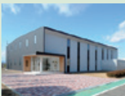
Exterior view of To-En-Ryo
