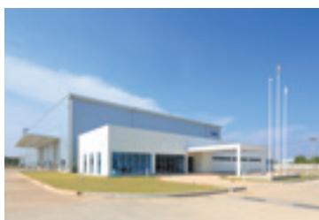
Thai casting plant A&M
